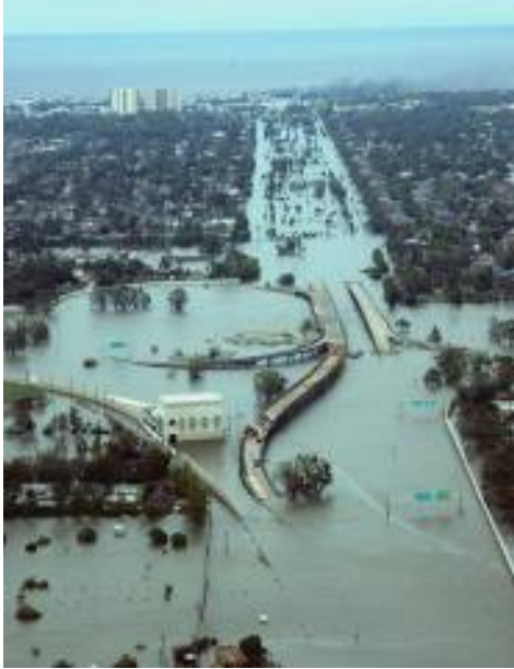
Figure 1. New Orleans infrastructure, underwater: Interstate 10 at West End Boulevard, view toward Lake Pontchartrain, August 29, 2005, shortly after the passage of Hurricane Katrina. U.S. Coast Guard photograph by Petty Officer 2nd Class Kyle Niemi.
